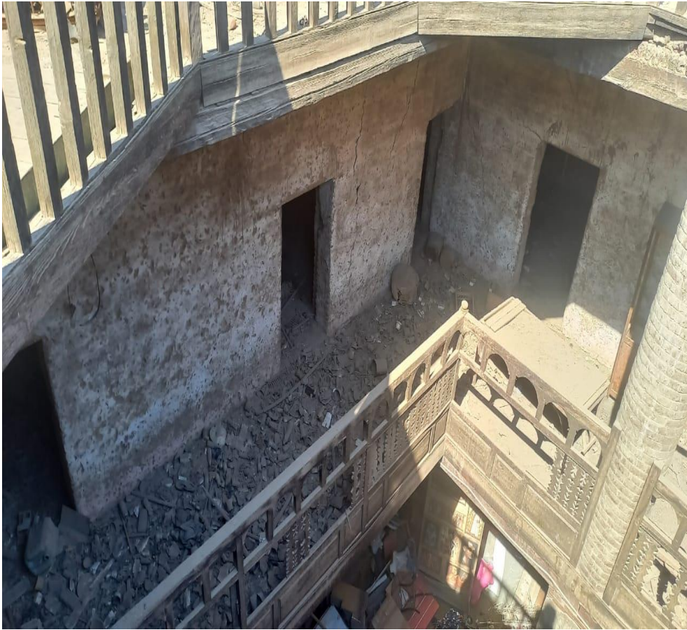
(Fig.4) using mud brick and qasmral in Wekala
