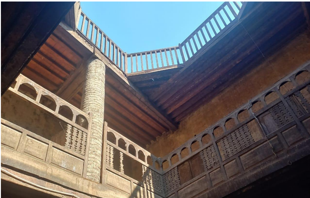
(Fig.8) using the palm trunks in ceiling and the malqaf for ventilation Source: taken by researcher
